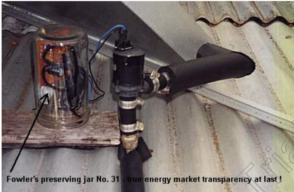
**Hiding under the heat-exchanger (solar collector) are the waterproofed Mini-Maximiser and the Davies,Craig brushless 12 V DC Electric Booster Pump**
